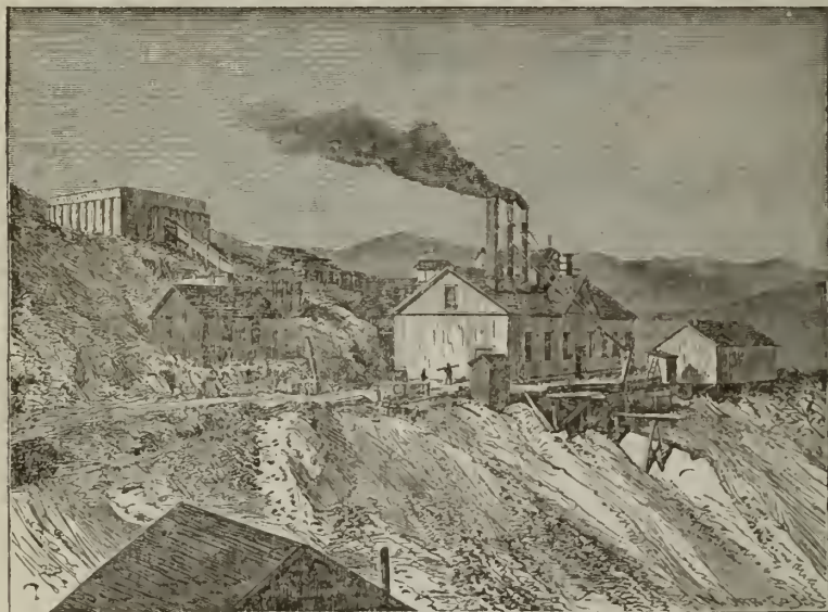
VIEW OF HOISTING WORKS AT SHAFT NO. 2, SUTRO TUNNEL.
